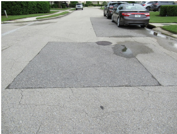
Asphalt pavement at 97 th Street East – large patches – Legacy neighborhood
