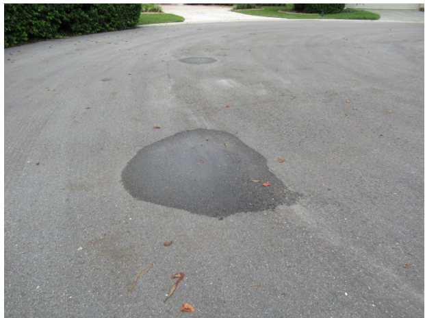
Asphalt pavement at 88 th Street East – depression and standing water – Legacy neighborhood
