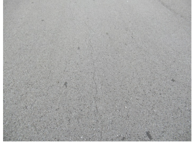
Asphalt pavement at 54 th Avenue East – cracks evident – Legacy neighborhood
