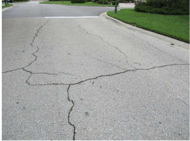
Asphalt pavement at 52 nd Avenue East – cracks evident – Legacy neighborhood
