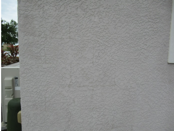
Cracks evident – north gate house
