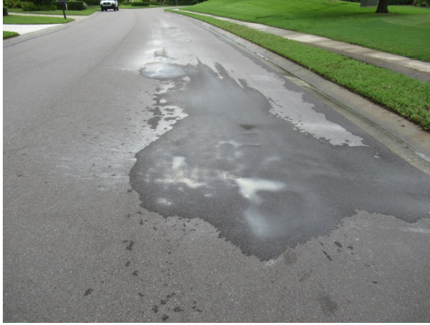
Asphalt pavement at 88 th Street East – subsurface water pumping evident - Legacy neighborhood
