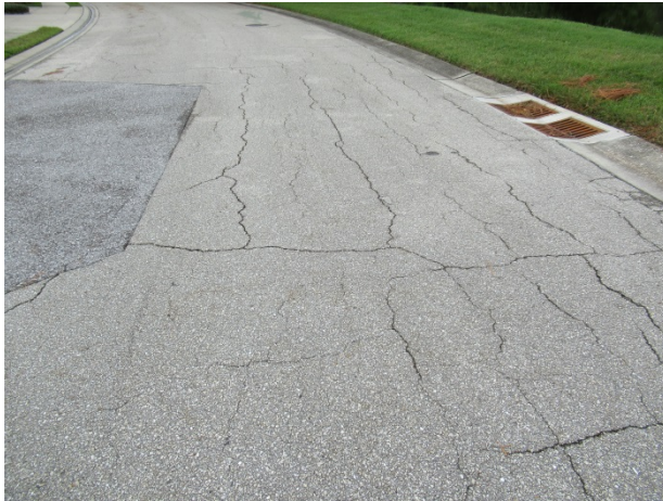
Asphalt pavement at 54 th Avenue Circle East – large patches and cracks evident – Legacy neighborhood
