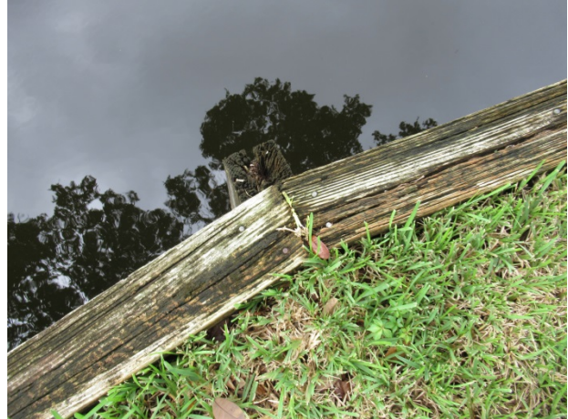
Deterioration of top rail
