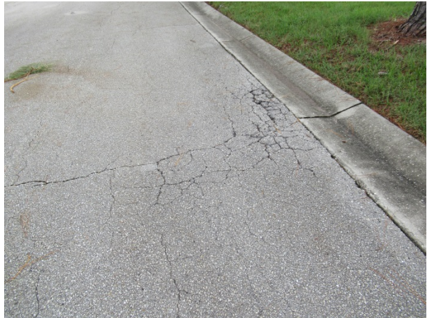
Asphalt pavement at 54 th Avenue Circle East – cracks evident – Legacy neighborhood
