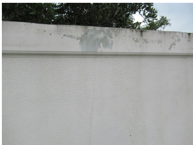
Paint deterioration and cracks – Links neighborhood
