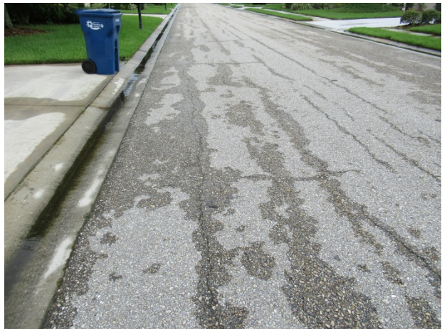
Asphalt pavement at 97 th Street East – numerous cracks – Legacy neighborhood
