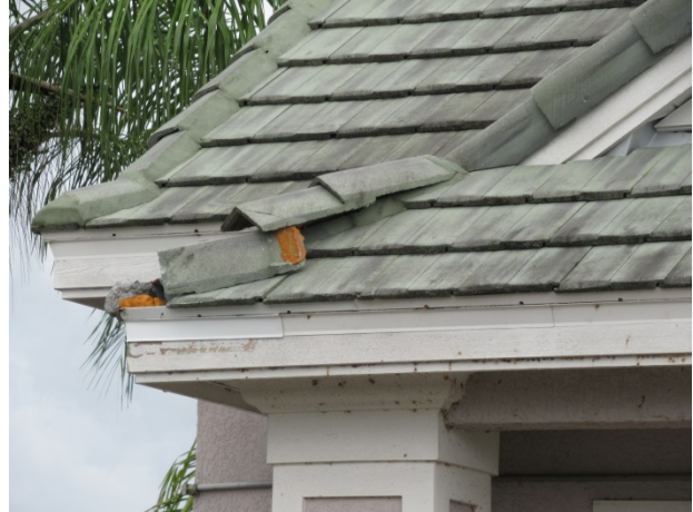
Damage due to vehicular collision
